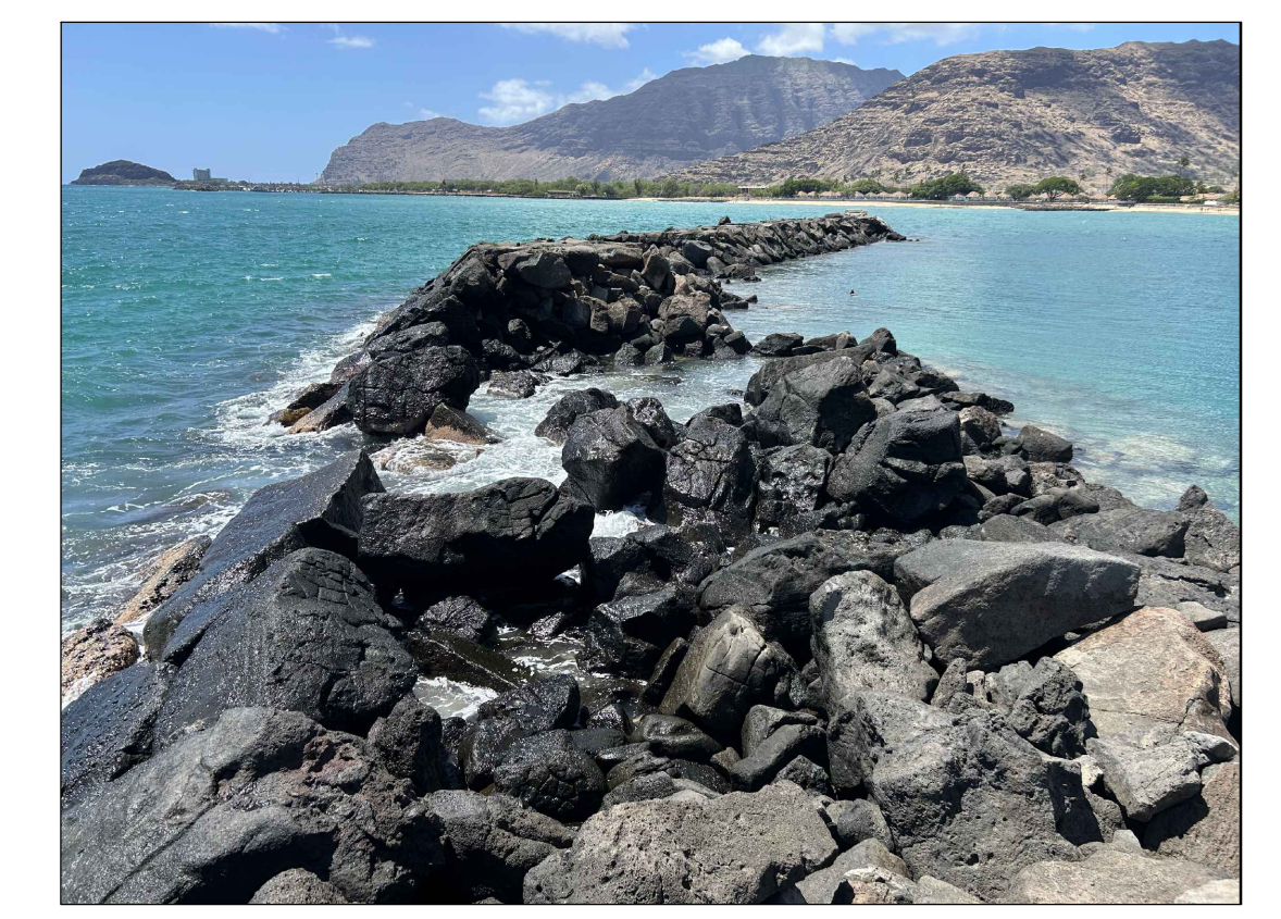
GROUND PHOTOGRAPH - SITE 3 APPROX. STA 5+25, LOOKING NORTH
