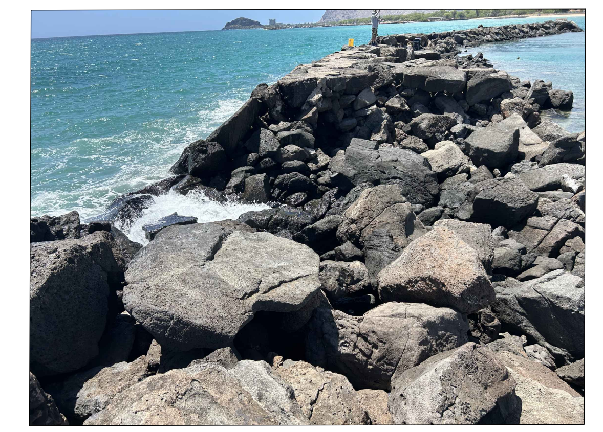
GROUND PHOTOGRAPH - SITE 2 APPROX. B STA 4+25, LOOKING NORTH
